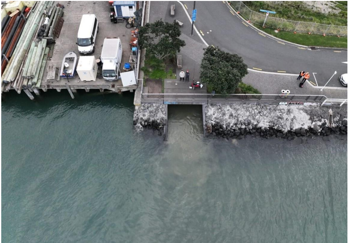
Figure 1 Footage of the sewerage overflow
